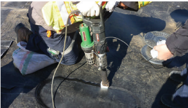
Extrusion Fillet Weld
